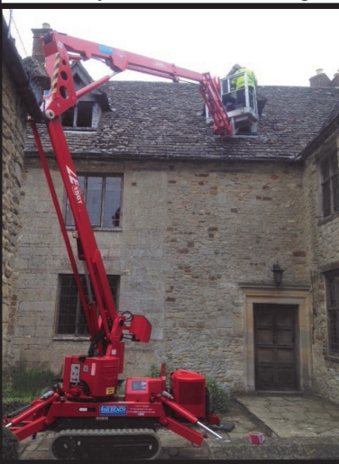
The last window being reinstalled after a year of repairs.
